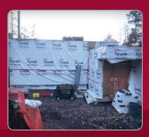
This residential construction site required temporary heat to dry the structure out and to help prepare it for insulation and drywall. The powerful fan drove the warm, dry air into both levels of the house and ensured a comfortable work environment.
