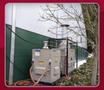
A winter craft fair moved into this tensioned fabric building requiring additional heat to ensure vendor and customer comfort. We added two hydronic heaters outside the building, supplying fan coils located inside creating an enjoyable experience for all.
