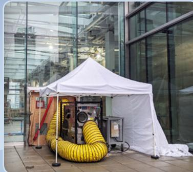
Humidity control through the final phases of construction is becoming more and more important. Contractors can deliver a building that has a balanced humidity level and can greatly reduce warranty work for drywall cracking, nail pops and other shrinkage problems.
