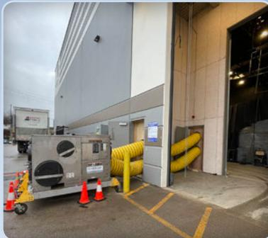
The heated pool for this film production produces lots of humidity. Left unmanaged, this moisture condenses on the structural steel of the studio and rains down on the production. Our desiccant dehumidifier kept levels in check and filming on schedule.
