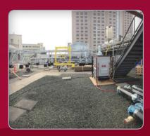
This hydronic heater took over the job of keeping ice and snow off of the helipad of Vancouver General Hospital during a renovation and upgrade project.
