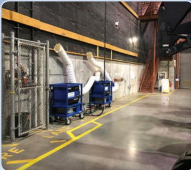
Whenever a film crew is shooting underwater, one of the major concerns is managing humidity levels in the studio. The massive swim tank is full of hot water and constantly evaporating. That excess humidity has the potential to condense on the studio's structural elements. When conditions are poorly managed this moisture rains down from everywhere and ruins the shoot.
