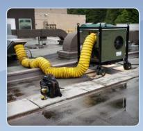
A quick response was required to keep the summer heat from ruining the plants in this botanical facility. Tying into the building ventilation system allowed for even distribution of the conditioned air. We located the unit on the buildings rooftop and kept any inconvenience to the public well out of the way.
