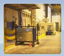
The MCC (Motor Control Room) in this plant suffered from excessive heat build up during the summer. An overheating problem would result in the control devices shutting down, placing the production in jeopardy.
