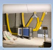
Temporary electrical vault cooling allowed this contractor to shed their temporary power and energize the building electrical vault.
