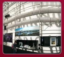
This event required large scale electric heating but also required this to be delivered with as little noise as possible. Our ducted solution allowed the unit to be located back of house. We were able to keep guests to this temporary structure warm and comfortable.
