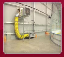
This large civic athletic centre is relatively un-heated. During a very cold winter our 60 kW electric furnace added just enough heat to make it comfortable. This sprung tent structure doesn't have any insulation so heating can be quite costly, unless it's done on as needed basis. Perfect fit for Cool Air.
