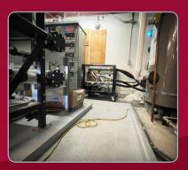
When this municipal boiler system failed, Cool Air provided a 1.2M BTU hydronic heater and a 1M non-potable heat exchanger. The heat exchanger provided the physical separation between the hot loop and the building loop.
