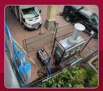
This potable application allowed the domestic hot water side of this residential building to stay viable during a planned shutdown. Residents had a reliable hot water source for cooking and showering. The stainless-steel heat exchanger is double walled and rated to be used in potable water applications, and we only release them to those very specific projects.
