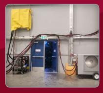
Another interesting use of our heat exchangers! This heating project was in an under-heated facility being used as an immunization centre. It required the use of only regular water running through hoses inside the space. We positioned our heat exchanger just inside the building, and ran glycol in the hot loop and clean water in the inside loop.
