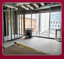
This construction site benefited from effective heat distribution. Six fan coils operated off of a single hydronic heater. The 200k BTUs of heat from each fan coil ensured that comfortable and dry conditions existed as the building transitioned into the finishing stage.
