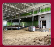
A temporary heating package was required during the construction of this large municipal pool project. A combination of 200k and 600k BTU fan coils was utilized to distribute heat evenly throughout the space.
