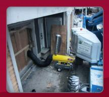
Small scale construction heating projects are a perfect match for this specialized heating unit. Separate combustion air allows for high temperature supply air but with a low humidity level. Dry air enables moisture trapped in construction materials to be released resulting in a drier project.
