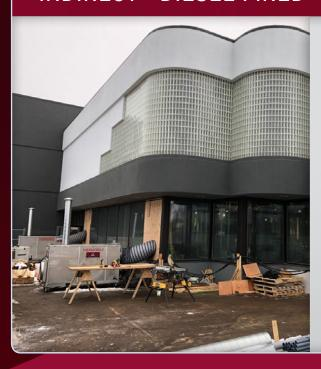
If you need major heat, then this is the equipment for you. Running on diesel fuel, they are well-suited for heating construction projects or temporary structures. Waste gases can easily be ducted to the outside if the unit needs to sit inside.
