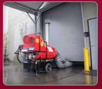
By placing the supply duct under the roll-up door, we were able to heat this warehouse simply and effectively with virtually no time spent on preparation or installation.
