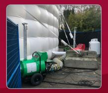
This yearly winter festival utilizes numerous unusually shaped temporary structures. This domed structure had openings in the base that allowed us to easily pass our duct work right inside. Perfect when cool temperatures make conditions inside uncomfortable.
