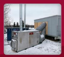
This senior's care facility required additional heat during cold weather, as they budgeted and planned for a system upgrade. This unit sat on the roof of the building and clean warm air was ducted into the existing ductwork plenum. The supplemental heat we provided ensured the residents were comfortable through the fall and winter.
