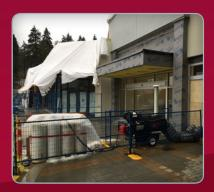
This mall upgrade included new mechanical facilities. When cooler weather moved in, management needed to keep shoppers comfortable. By utilizing this temporary access opening and building a safety barrier around the unit, we were able to provide warm, clean air into the building.
