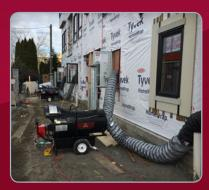
Multiple units were required to keep this condominium project warm and dry through the construction process. Warm interior conditions allow construction schedules to move forward as planned, give a better finished product, and reduce call backs for shrinkage and drying issues.
