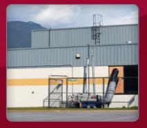
While the dedicated boilers and air handling units were being replaced, these natural gas fired units provided temporary heating for this community centre.
