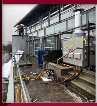
Whether you need to temporarily replace an existing boiler or you have a complex heating application that requires a high degree of customization, this unit is the one for the job. This hydronic heater requires a fuel source from either a large propane cylinder or direct natural gas hook-up.
