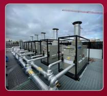
This large scale mall expansion and renovation project required a 4 year commitment to provide a heating and cooling equipment plant. Five 1.2M BTU Hydronic Heaters ensured that the remaining facilities that housed clinics, offices, residential tenants and commercial space had the heat and hot water they required to operate without interruption.
