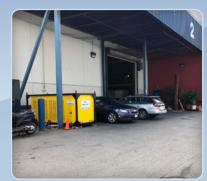
This 30 ton chiller was located outside a film stage. Relatively small and compact, it was quiet enough to run when they were recording sound. A closed loop of hose connected the chiller to one of our air-handling units inside. Flexible ducting easily directed the conditioned air to wherever it was needed.
