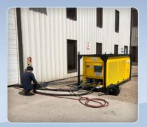
When temperatures inside this manufacturing facility began to affect productivity levels, this 30 ton chiller and our matching 30 ton air handler were brought in to restore temperatures inside the plant to acceptable levels. Once the conditions improved, so did morale and output. When fall weather brought cooler outdoor temperatures, we removed our gear.
