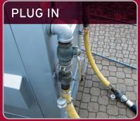
2" camlock hose fittings can carry water or a glycol/water mix to your building's dedicated loop or to our portable fan coils, whichever is more convenient.
