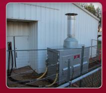
When this building's boiler needed an upgrade, we stepped in to ensure they'd have heat while the work was being done. Our unit hooked into their existing water/glycol loop, for a quick and painless install.
