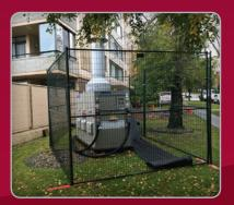
This ten storey concrete tower lost its heating when a flood wiped out its boiler. Quick response by Cool Air meant this replacement hydronic heater was installed and operational in a little over one day.
