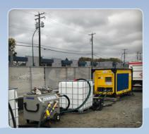
Concrete generates large amounts of heat while curing, a process known as hydration. Installing embedded cooling lines prior to pouring allows us to circulate chilled water throughout the slab and strip the heat away in a controlled manner. This 30 ton unit coupled with a 1000 litre tote ensured the curing process was successful and without issue.
