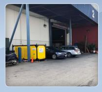
This 30 ton chiller was located outside a film stage. Relatively small and compact, it was quiet enough to run when they were recording sound. A closed loop of hose connected the chiller to one of our air-handling units inside. Flexible ducting easily directed the conditioned air to wherever it was needed.
