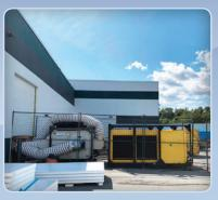
This food manufacturer was expanding quickly and to keep up with consumer demand, they needed to install more ovens. This added heat load inside their plant made the workers uncomfortable and impacted the quality of their product. We paired a 60-ton chiller and 50-ton air handling unit outside their overhead door. This powerful combination pulled the hot air from the manufacturing facility outside, while returning cool, fresh air into the facility.
