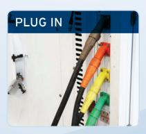
4" chiller hose ties easily into our air handling unit and just as simply can tie into your building loop, or one of our portable chillers.
