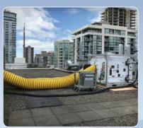
This 50-ton air handling unit provided temporary cooling for the radiology department at a local hospital. The unit was hoisted onto the rooftop, while they replaced their cooling coils. Once the changeout was complete, and they finished commissioning and testing, we removed our equipment and the site was returned to normal.
