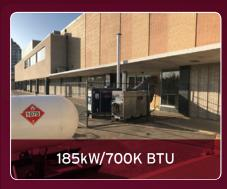
This large Calgary furniture store lost all of its heating just as the weather turned cold. We had a display windowpane removed, installed a filler panel, and supplied the store with warm glorious heat. Once the contractor repaired the boilers, we rolled up our gear and left the site looking like we had never been there.
