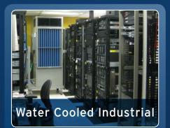
We deployed our water-cooled units for this server room. This custombuilt portable technology is unique. The heat energy is rejected into the building's chilled water loop or domestic water system. These units are extremely effective when the server room or data centre is located deep inside a building.
