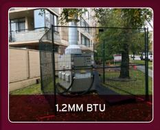
This 10-storey residential tower was without heat after a boiler failure. With cooler temperatures on the horizon, building management realized a temporary boiler was required to keep tenants comfortable until the replacement boiler was operational.
