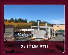
The boiler for the Amazon Jungle exhibit had reached its life expectancy and needed to be replaced. Our temporary 2x 1.2MM BTU hydronic heaters took over heating the air and water for 10 weeks, while the removal and re-installation of the new boilers took place.
