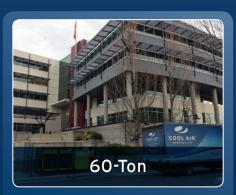
This 60-ton chiller was required to cool this building while the roof-top mounted chiller was being replaced. The chiller hoses and the power feed were run up the outside of the building and tied into the building loop at the roof-top level. Fencing protected the public from walking into the area.
