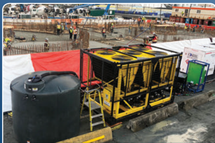
Concrete Slab Cooling
