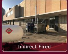
This large Calgary furniture store lost all of its heating just as the weather turned cold. The natural gas feed was too far away so the decision was made to use propane instead. We had a display windowpane removed, installed a filler panel, and supplied the store with warm, glorious heat. Once the contractor repaired the boilers, we rolled up our gear and left the site looking like we had never been there.
