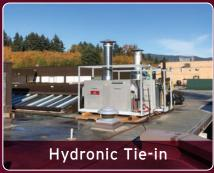
The boiler for the Amazon Jungle exhibit at the Vancouver Aquarium had reached its life expectancy and needed to be replaced. We supplied a dual 1.2MM BTU hydronic heating package to heat the exhibit's air and water, allowing the contractor the peace of mind to remove the old boiler and install the newly procured boiler package over a ten-week duration.
