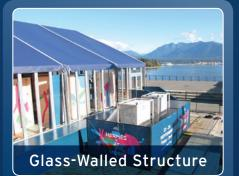
Hermes set up this large temporary structure in downtown Vancouver to showcase their products and craftsmanship. These units heated and cooled the structure for four weeks. The elevated deck allowed us to duct our conditioned air under the structure and into the space through diffusers we installed in the floor.
