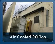
These air cooled units are designed to sit out in the elements. They can be ducted on both the supply and return air side. Local or wired remote control allow for complete temperature control or simply flat out cooling. A very versatile electrical vault cooling unit.
