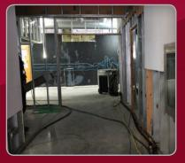
This construction project required temporary heat through the winter months. Our hydronic heater delivered a constant flow of hot water to these fan coils located inside the areas under renovation. This warm environment greatly reduced the wait time between drywall mudding and painting recoats.
