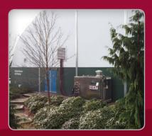
This structure hosts a Christmas Craft fair every December. It is normally under-heated and therefore not warm enough to keep vendors and their customers comfortable in cold weather. This hydronic heater was installed to distribute hot water to fan coils located inside the structure.
