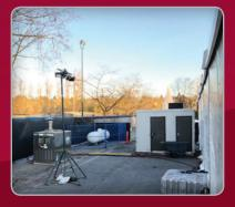
The versatility of this hydronic heater allows it to be placed outdoors adjacent to structures to deliver hot water into the space. We can tie into the existing piping or provide fan coils to distribute the warm air in the
