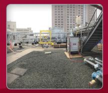
This hydronic heater took over the job of keeping ice and snow off of the helipad of Vancouver General Hospital during a renovation and upgrade project.
