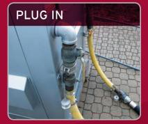
2" camlok hose fittings can carry water or a glycol/water mix to your building's dedicated loop or to our portable fan coils, whichever is more convenient.
