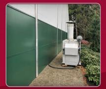
It was simple to place this boiler back behind the building, out of sight and out of the way of customers. We hooked up to our client's natural gas line and fired up the boiler. Warm conditions made everyone happy.
