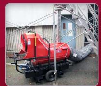
Exterior wall repairs in the winter bring temperature control issues. This diesel heater running on a thermostat maintained conditions that allowed the stucco finish to properly cure.
