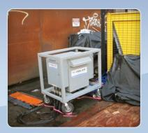
This transformer was used at a film set to energize one of our 60-ton chillers. Set cooling is critical during summer months to keep cast and crew cool despite all of the lights and equipment.
