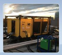
When this building's chiller required maintenance, Cool Air provided a temporary chiller. With only 600 volt power available we provided a packaged portable transformer to step down the voltage and energize the chiller.
