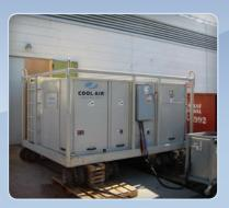
This large telecom space required our auto transformer to facilitate energizing this 25 ton air conditioning unit.
