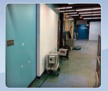
This building needed temporary heat during renovations; 208 volt power wasn't available in this area but 600 volt power was. Our portable transformer was the simplest solution.
