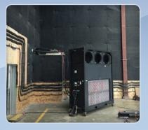
Placed inside a film stage with multiple setpieces used at different times in the day, this air handler unit is ready to supply spot-cooling to specific areas as needed.
