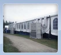
These units are made to sit outdoors and can handle variable weather conditions when operating in either cooling or heating mode. Three 20 ton units were called upon to manage the temperature and humidity levels and ensure that conditions were comfortable inside this Golf Canada venue at the RBC Canadian Open.
