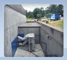
BC Institute of Technology holds its final exams every May in the school gymnasium. Complaints of uncomfortable conditions led the Facilities department to contact Cool Air for a viable solution. We positioned two 20 ton units outside the exit doors without compromising egress safety. Conditions inside were markedly improved and the quiet operation of our equipment meant the exam process went ahead seamlessly.
