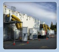
Three 20 ton units were required to maintain acceptable conditions inside this telco hub during a power infrastructure upgrade. Cool Air handled not only the temporary cooling requirements but the power distribution and power generation necessary to run this project.
