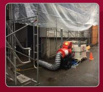
At this site, a lower level of continuous heat was needed to keep the stucco warm enough to cure. Luckily, the fuel tanks are compatible with our smaller 50 kW heaters, in addition to the larger 117 kW units.
