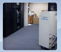
This was another example of what this versatile performer can handle. A shutdown of the server room unit required an equally sized temporary unit to take over the cooling load. Once the building system was operational, we simply rolled our unit out the door.
