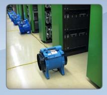
These Force 9 and Vortex Axial fans worked together to keep air circulating down these server aisles. Without the help of Cool Air, this room would have shut down from over-heating and phone and internet service would be interupted for thousands of customers.
