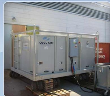
This large telecom space required our auto transformer to facilitate energizing this 25 ton air conditioning unit.
