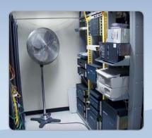
This server room needed increased airflow to ensure continuous operation. This pedestal fan was brought in to assist in the cooling process by driving more air through the servers.
