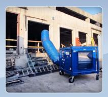
Construction sites often require extra ventilation during various stages of the project. This Hurricane was used to provide ample fresh air to workers inside while welding gases and exhaust fumes were present.
