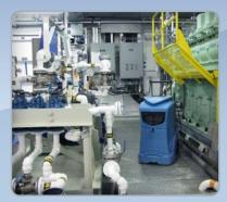
This dehumidifier was installed to control moisture in a sensitive area of this ship. Without the use of this unit, normal operation and maintenance would have been adversely affected.
