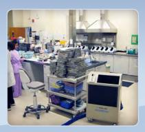
An undersized cooling system meant that this lab was uncomfortable in the summer. The supplemental boost provided by this unit ensured both heat and humidity were held in check. By properly managing the indoor air conditions, efficiency and productivity can match expectations.
