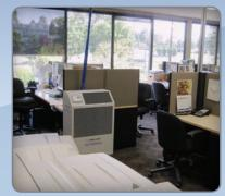
When this building system failed at the peak of a heat wave, four of these 1.5 ton portables were installed and comfort levels were restored. This was an ideal application for a premium portable unit.
