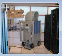
Fitted with the alternate 90° plenum, this 5 ton directed its full cooling strength at the server cabinet.
