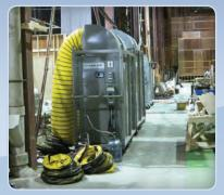
Large scale productions generate a huge amount of heat from the lights they use. Filming in large insulated studios traps the heat and humidity creating uncomfortable or even unbearable conditions. Multiple units such as these process the heat and make conditions manageable.
