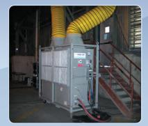
This industrial facility had its dedicated cooling system down for maintenance. Problems with parts meant the week that the project was planned to take, turned into a month. This 20 ton handled the heat more effectively than the building system, and when the job ended, we simply rolled the gear out the door.
