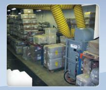
This warehouse was unbearably hot during the summer months. Installing a dedicated system was not cost effective so this 20 ton unit was brought in for four months. It kept the facility nicely cooled so that the staff could hide in the racking and sleep.
